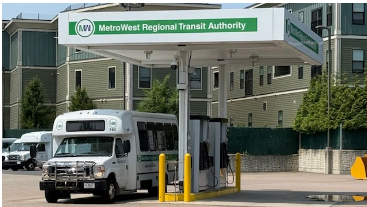
Figure 1. MWRTA Compressed National Gas Facility at Blandin Hub
